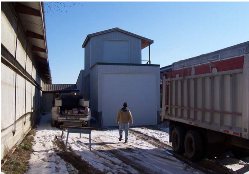
Manure Separator Facility
